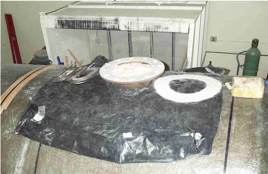
The rings are “painted” on to the cryostat opening using the same laminating resin that was used to adhere the cotton filter pads.
