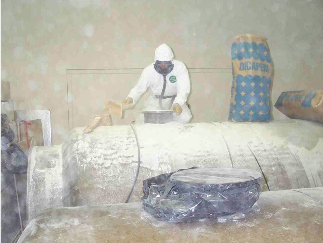
The perlite is spread inside and packed tight with wooden sticks that have flattened end-pieces. The full weight of Andy Zawacki can be brought to bear on the packing.
