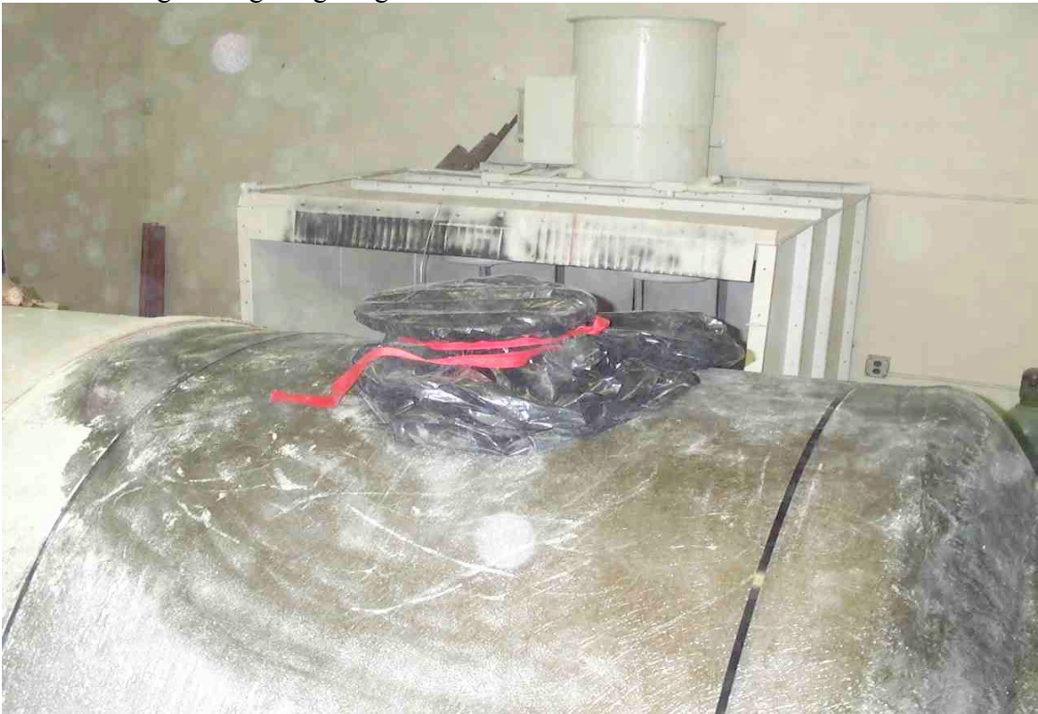
With perlite nearly to the top of the filter opening, the hold is then again protected with moisture using a tied garbage bag.
