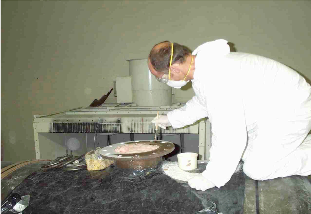
Pink insulating “wool” is packed against the perlite to prevent the perlite from plugging the filter. The edges are painted with laminating resin for adherence of the fiberglass “cloth” rings.
