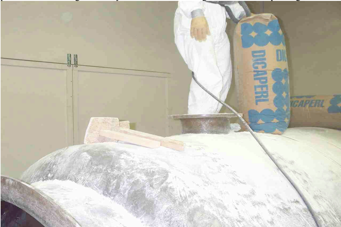
The perlite is spread inside and packed tight with wooden sticks that have flattened end-pieces. The full weight of Andy Zawacki can be brought to bear on the packing.
