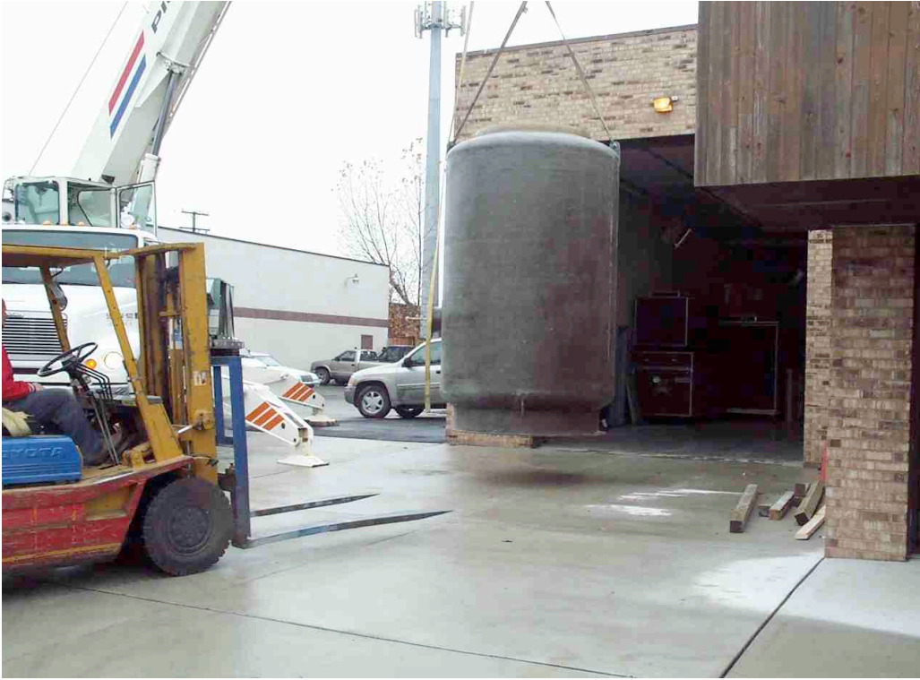
One in a vertical position, the cryostats can be placed on a forklift (pink insulation board used for padding) and returned to the warehouse for positioning.
