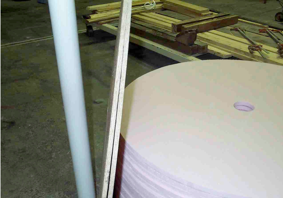
A plastic cylinder is inserted into a hole made in the middle of the pink insulation boards. Plastic rods through the insulation boards and plywood secure the insulation boards.
