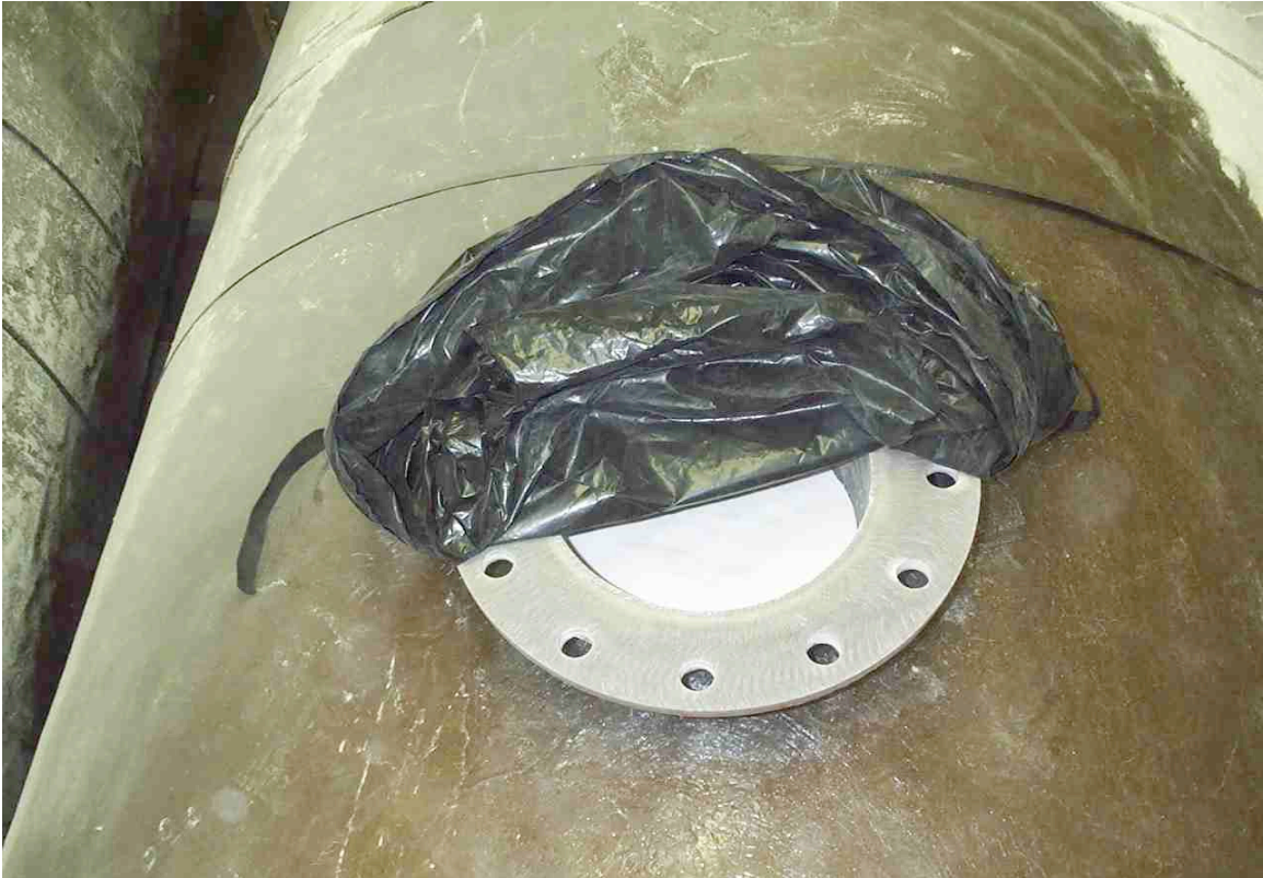
With perlite nearly to the top of the filter opening, the hold is then again protected with moisture using a tied garbage bag.
