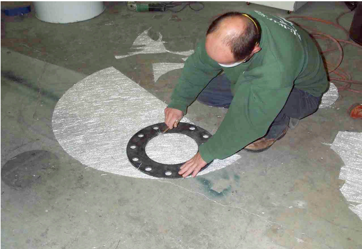
Rubber gaskets that were under the fiberglass lids on the filtration hole during shipment from New York are used as templates for cutting fiberglass “cloth” rings.
