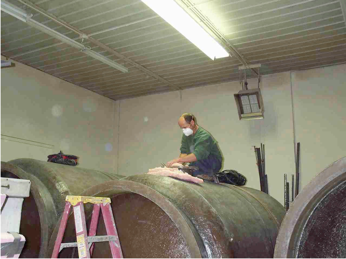
Pink insulating “wool” is packed against the perlite to prevent the perlite from plugging the filter. The edges are painted with laminating resin for adherence of the fiberglass “cloth” rings.
